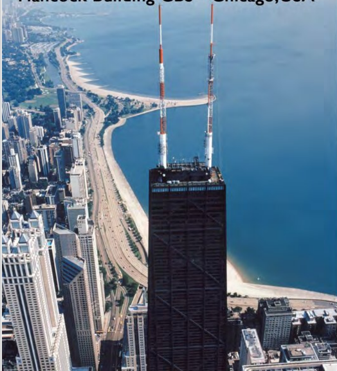
First DTV Antenna on the Hancock Building CBS - Chicago, USA
