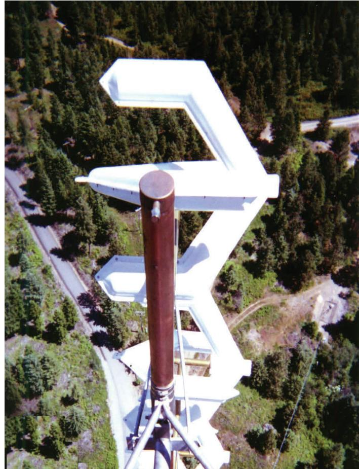
This antenna is designed with the same principles as JAMPRO's patented PENETRATOR series of FM antennas, which set the industry standard for FM side mount antennas. Optional 6-1/8" Center Feed available for higher power handling. The shunt fed design eliminates the need to "slug tune" the antenna in the field for optimum performance. Unlike similar, older designs, the Optimizer uses low impedance bays for un-excelled stability and band pass.
