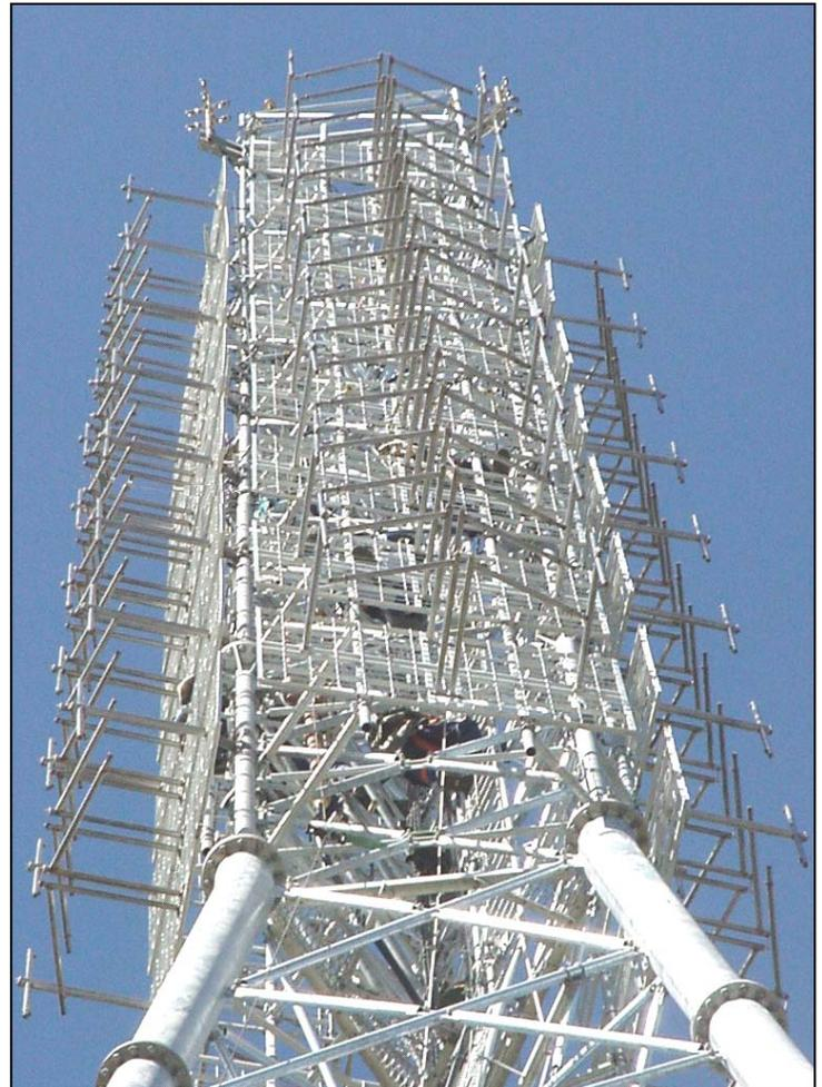
The design of this circularly polarized antenna may be configured to include varying levels of vertical polarization, with results ranging from small amounts of elliptical polarization to full circular polarization.
